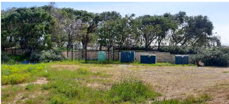
Cleared site with access to utility services
